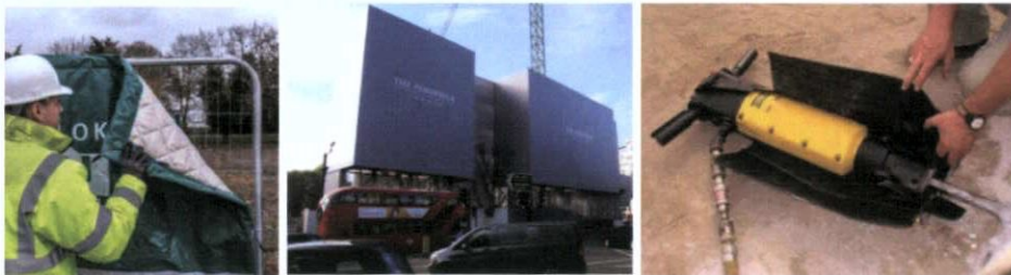
Figure 25 – Typical Noise Mitigation Measures
