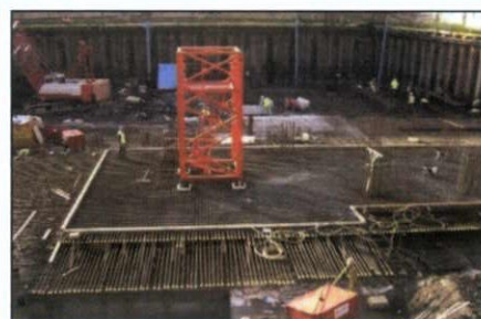
Figure 7 Typical Tower Crane Anchors
