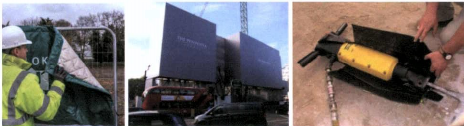
Figure 26 – Typical Noise Mitigation Measures
