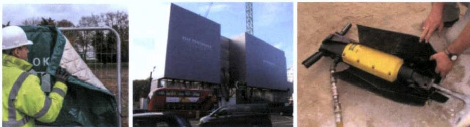
Figure 39 – Typical Noise Mitigation Measures
