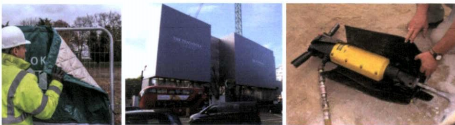
Figure 15 – Typical Noise Mitigation Measures
