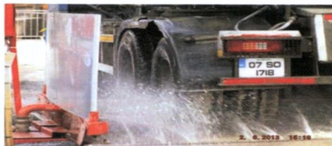
Figure 8 – Typical Wheel Washing Facility
