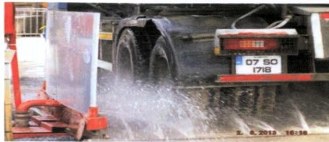
Figure 8 – Typical Wheel Washing Facility
