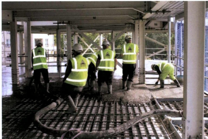
Figure 17 – Typical Concrete Pour on Metal Decking
