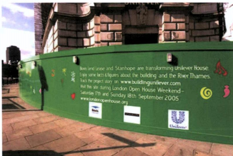
Figure 5 – Typical pavement hoarding with street lighting
