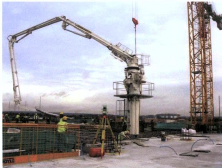
Figure 15 - Typical Concrete Placement
