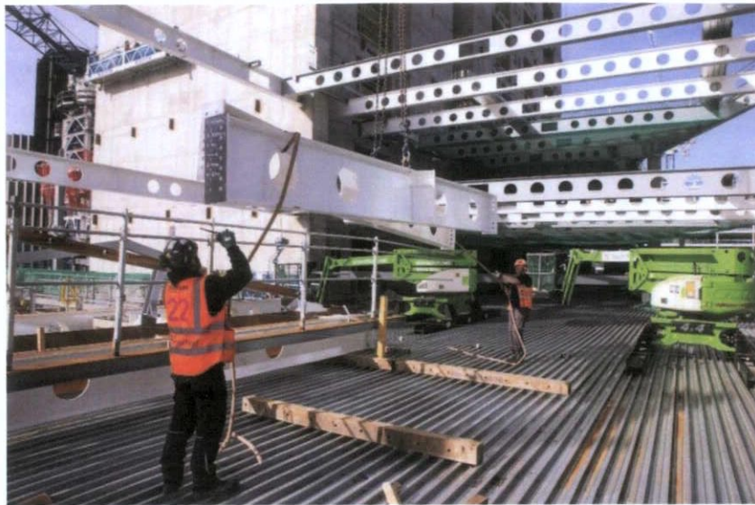
Figure 16 – Typical Steel Frame Erection
