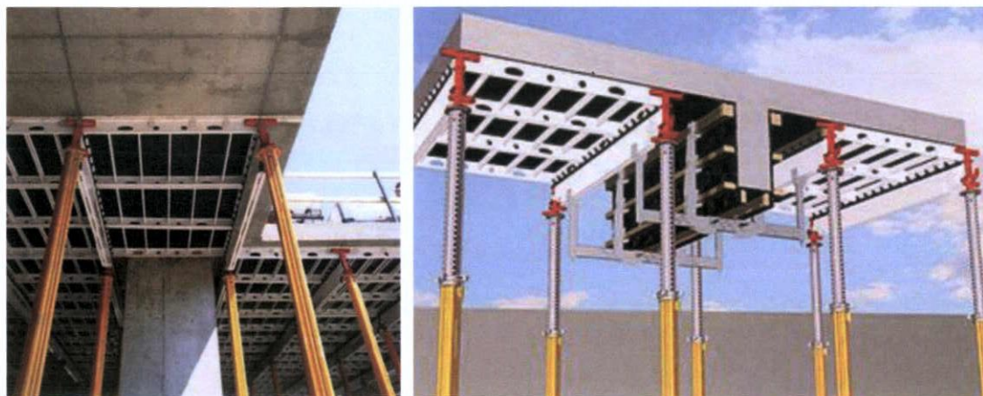
Figure 14 - Typical RC Formwork (Skydeck)
